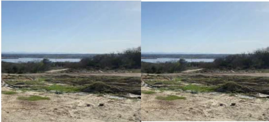
Figure 66: Different views of Dharabi Dam, Chakwal
