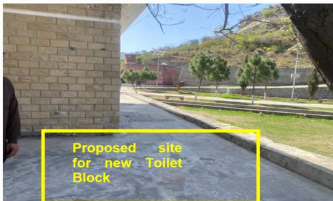
Figure 80: Proposed site for new toilet block at TDC Kartas Raj, Chakwal
